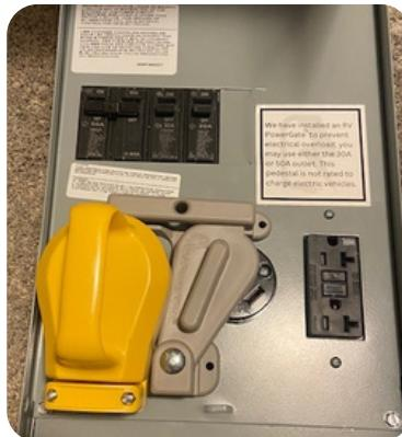
Remove white dot sticker backing and dry fit PowerGate around a 50A plug. This will ensure proper alignment.
