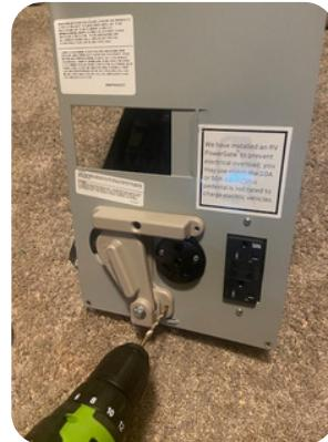
Remove face plate of pedestal and drill four screw holes through the faceplate
